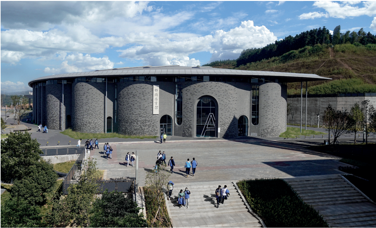
Tianhua designed a gymnasium and pool for Fujian Jian'ou First High School in Jian'ou City, Fujian. Sitting at the foot of Tianhu Mountain, it creates a visual focal point at the entrance to the campus and its form is inspired by two leaves
